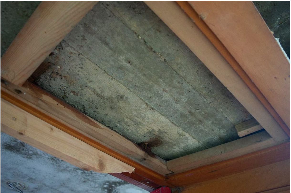
Plate 16: Board-marked cast concrete forming the lintel of the doorway into the children's library from the link corridor (NAC21-0048).
