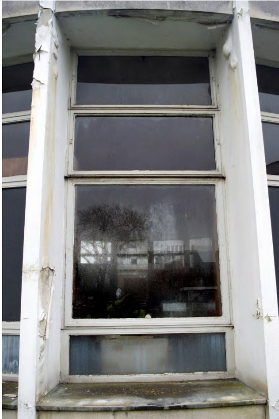
Plate 5: An example panel showing glazing with concrete mullions to each side (NAC21-0099).
