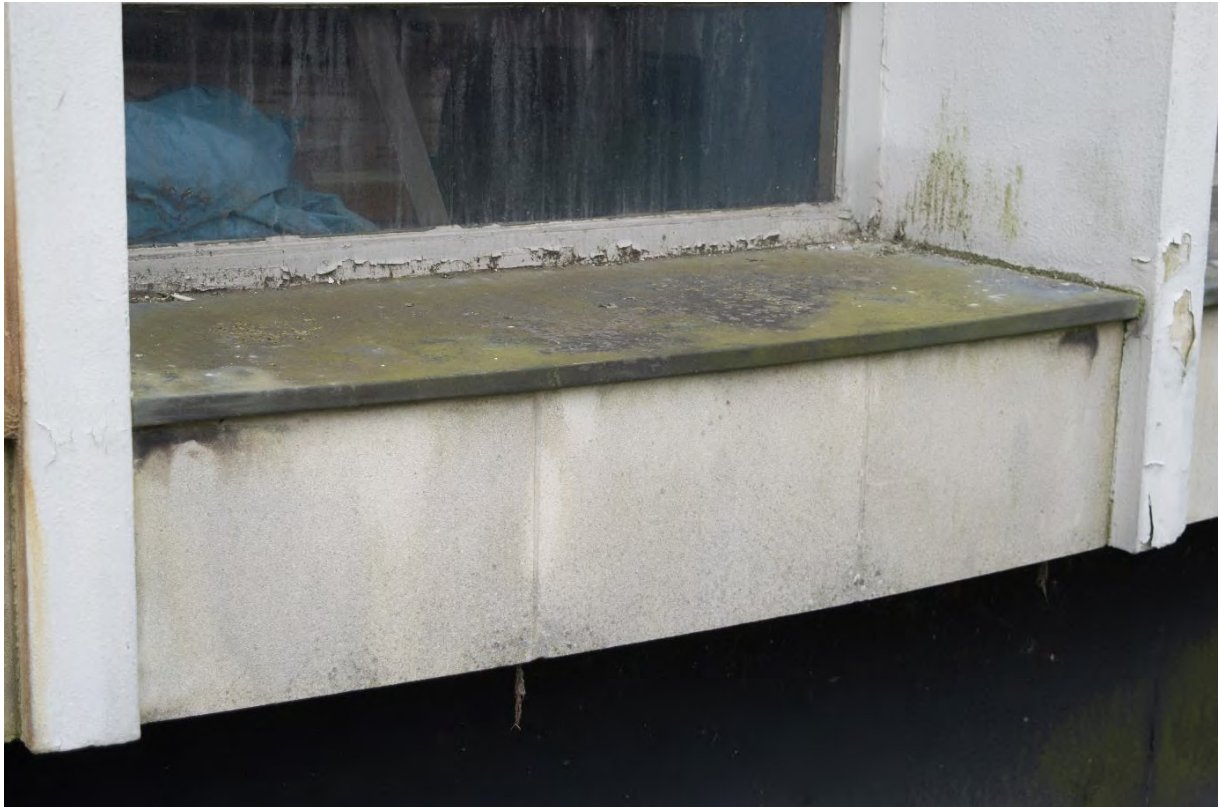
Plate 6: An example slate sill (NAC21-0101).
