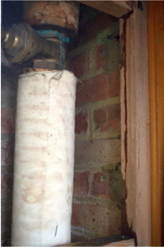
Plate 15: Exposed Fletton brickwork seen in the link corridor (NAC21-0051).
