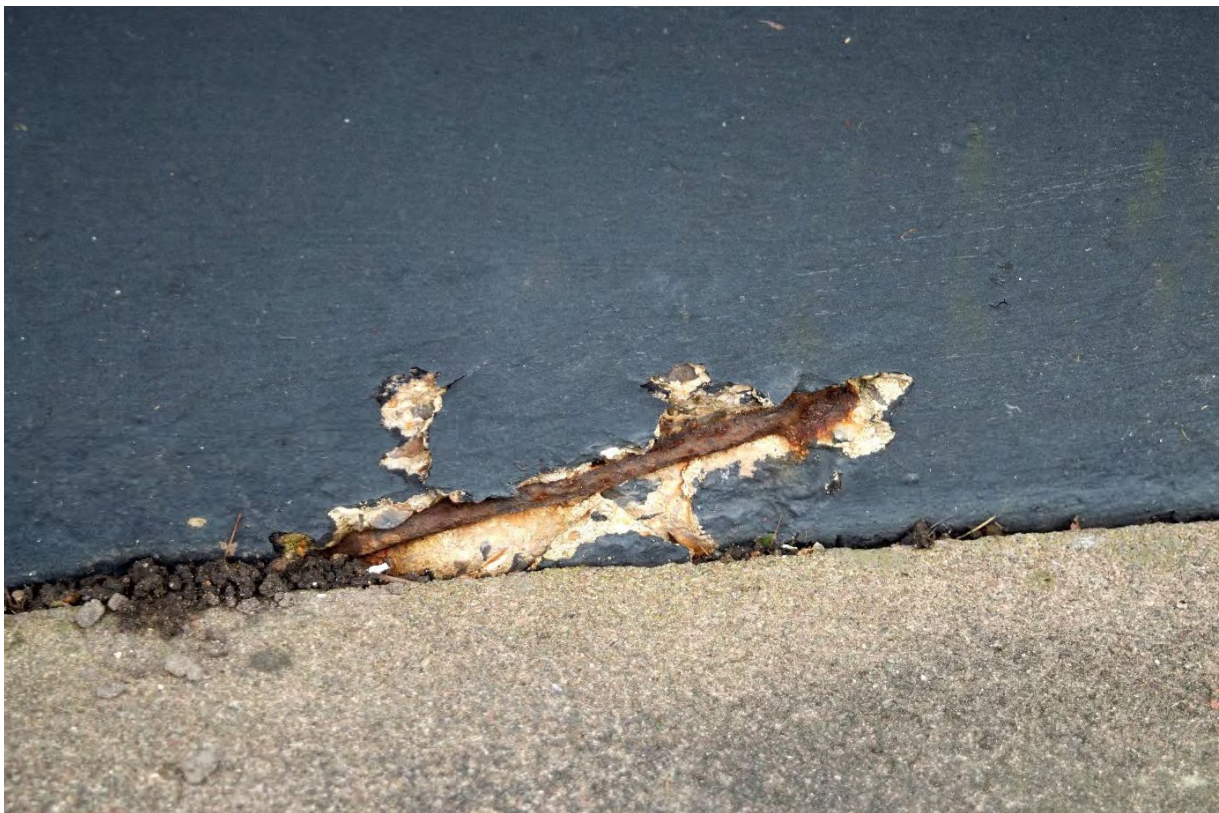
Plate 4: Detail of reinforcing bar in the plinth (NAC21-0096).
